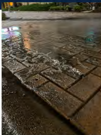
Old Sealer Melts and Lifts off Pavers and Concrete
